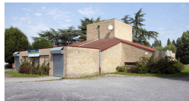
Élévation sud est. Phot. Pierre Thibaut IVR31_20155900718NUCA
