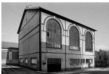
Chaufferie, flanc sud. Phot. Francis Dubuc IVR22_19908001105Z
