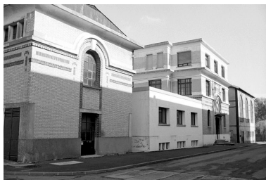
Bureau, chaufferie. Phot. Francis Dubuc IVR22_19908001110Z
