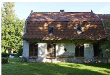
Façade sud. Phot. Delphine Volto Jourdan IVR32_20245903087NUCA
