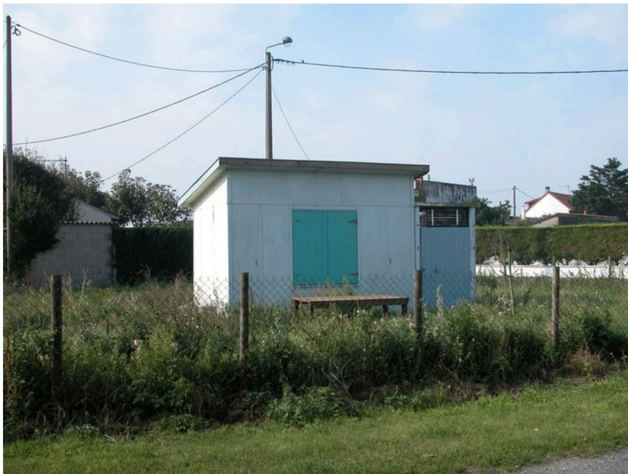
Bungalow, rue de Bougainville (1988 AY 175).
