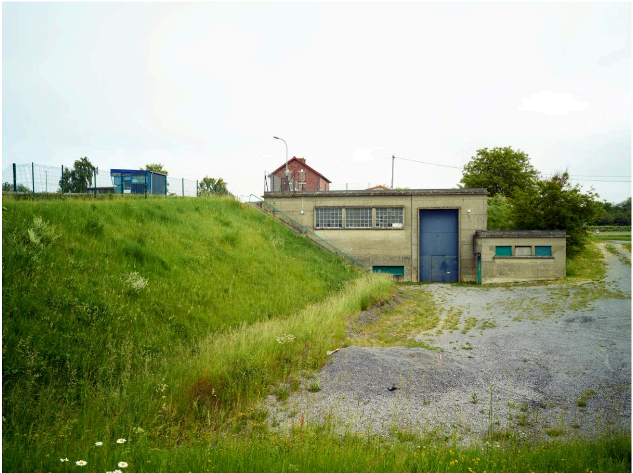
La station de pompage.
