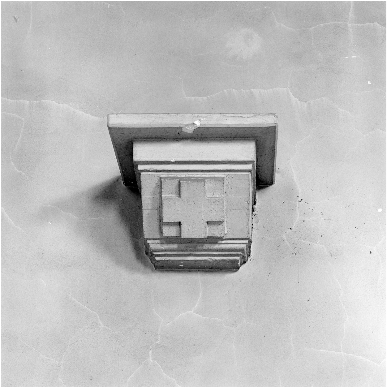
Chapelle, transept ouest, console.
