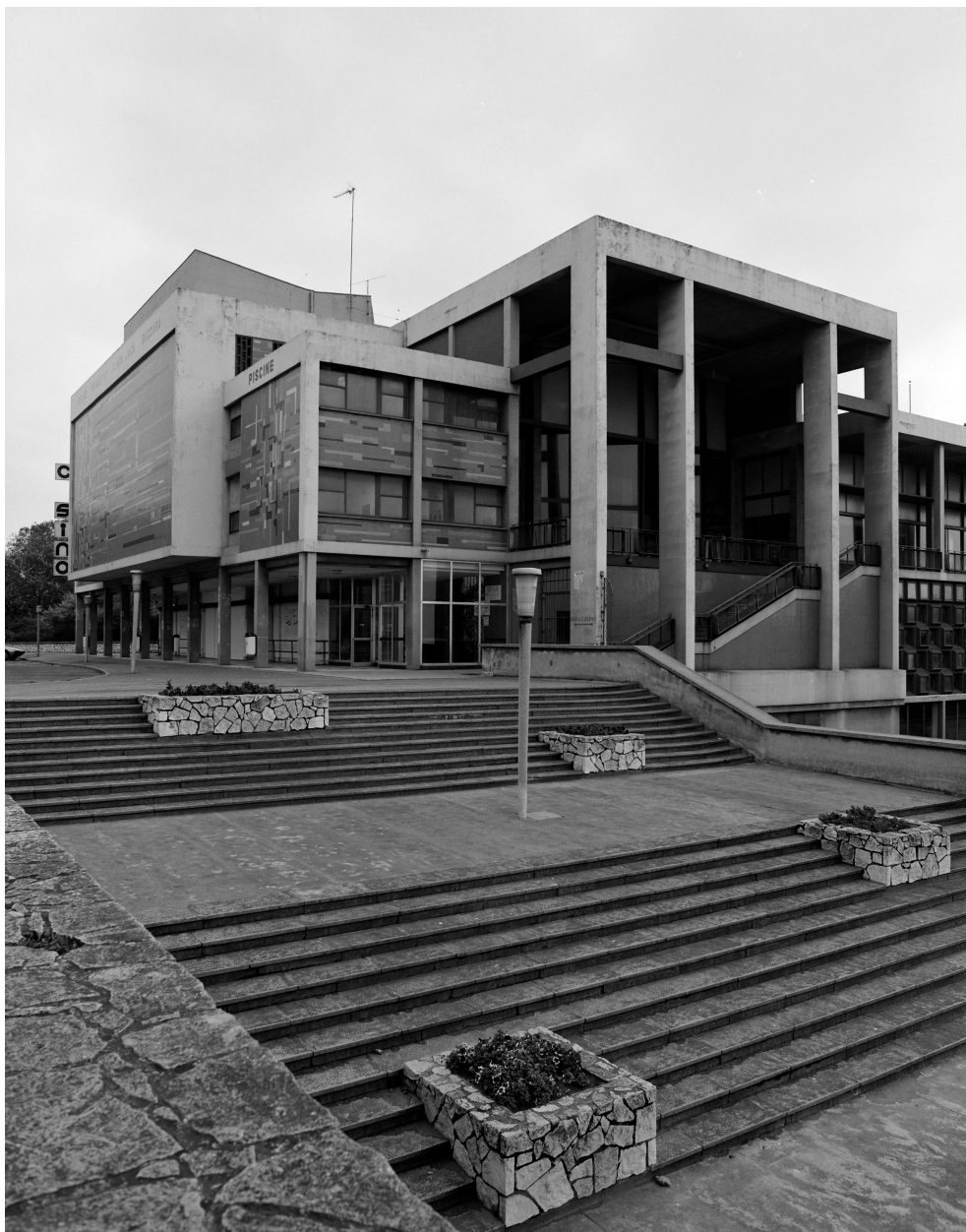
Casino municipal, angle nord.
