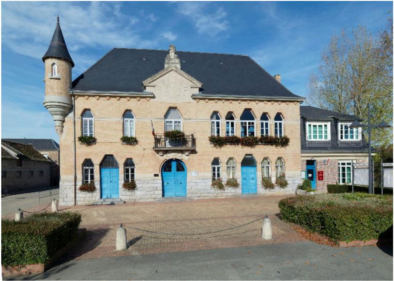
Façade principale de face.
