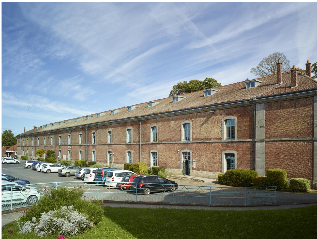
Caserne Lowendal, façade principale.
