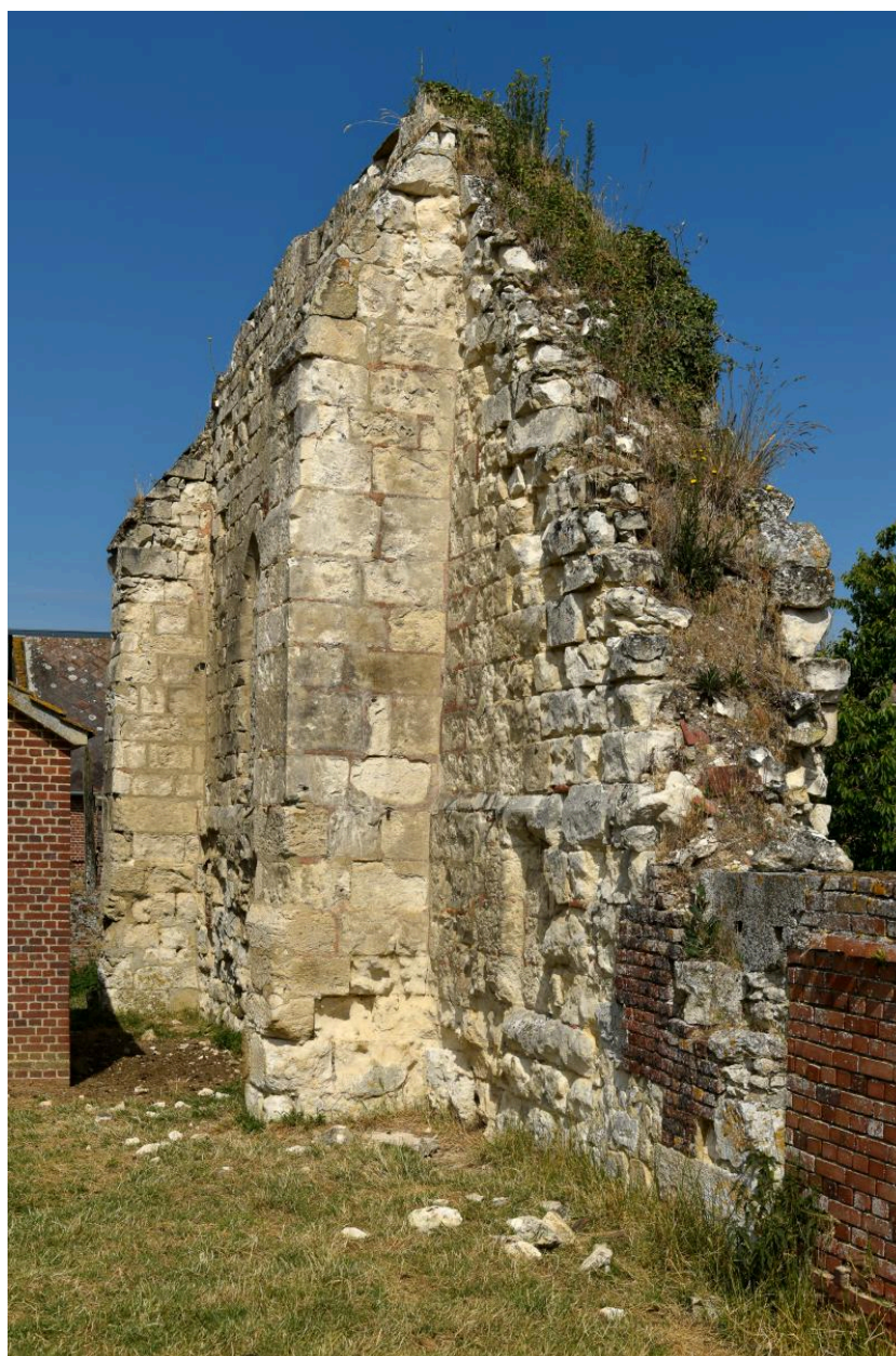
Pignon sud : contreforts.
