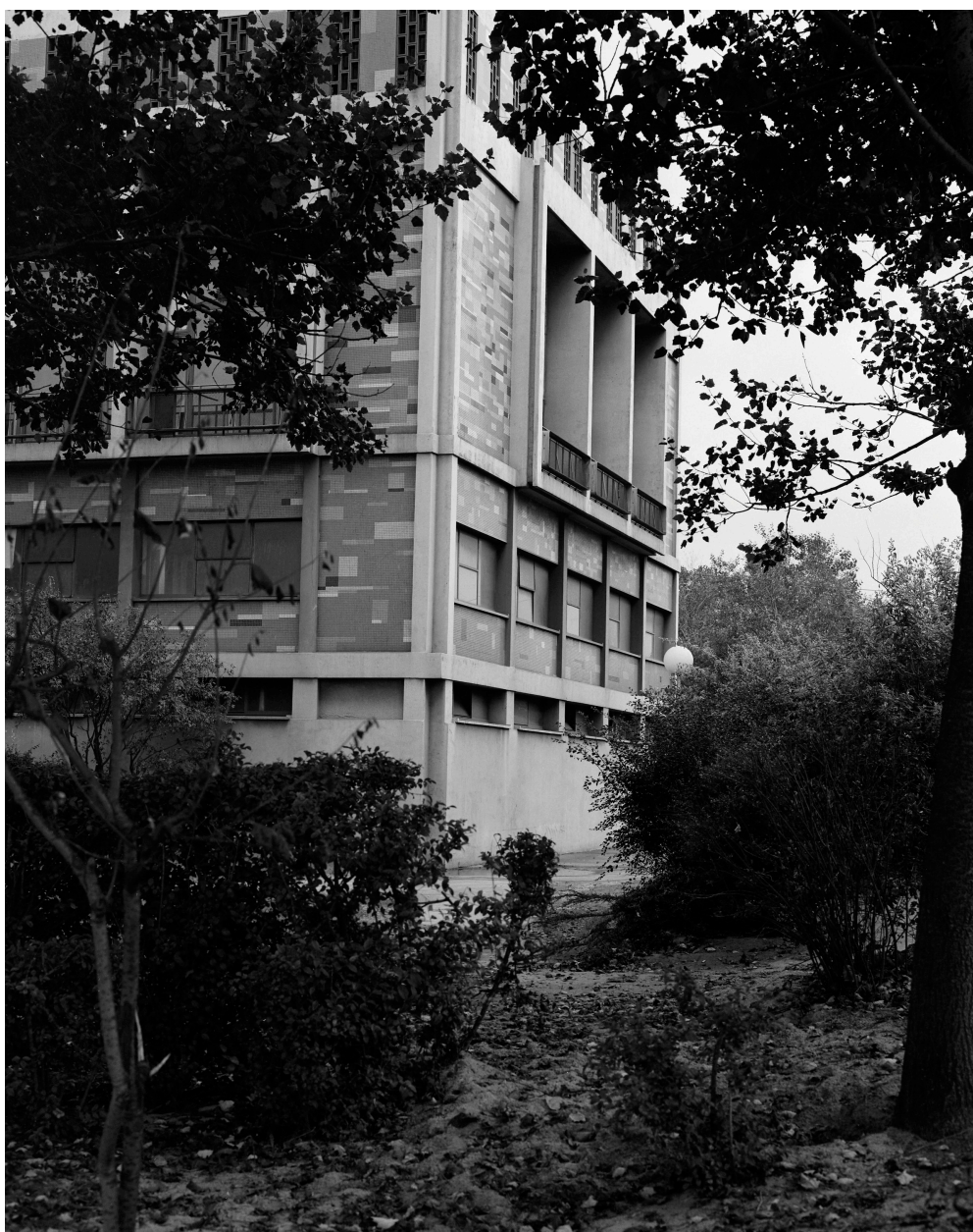
Casino municipal, pignon sud.
