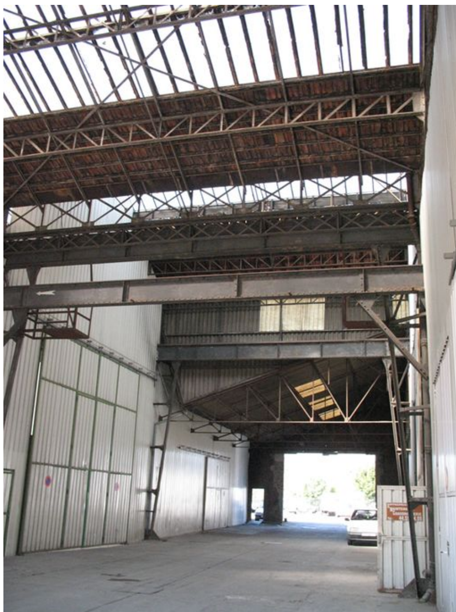
Structures des charpentes.
